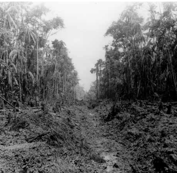
Photo 2.5. and Photo 2.6. Extensive stands of Virola surinamensis (Roland.) Warb. (Myristicaceae), in the coastal swamps were opened up by small canals. In the early days these canals were sprung with dynamite, but later they were dug out with machines. (Photo J.H.A. Boerboom)
